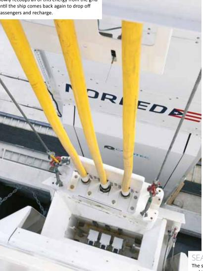
he Ampere was developed from the ground up as an electrically powered vessel, made exclusively of aluminum. With three battery packs, one on board and one at each pier, the ferry only uses 150kWh per route, which corresponds to three days use of electricity in a standard Norwegian household. Siemens developed the ferry's drive system and put up charging stations with lithium-ion batteries, which are charged from renewable energy, namely hydro power.
